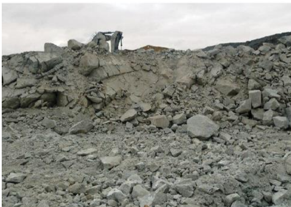
Figure 1.2. Visible rock formation after blasting
